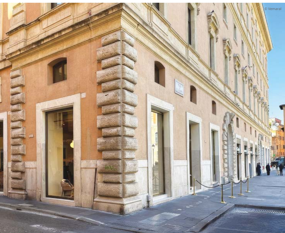
Modern powder-coated window frames on a historic Roman façade.
