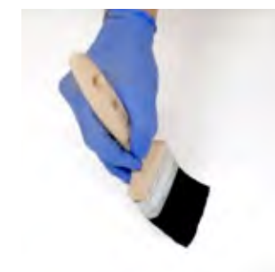
SEALING AND PROTECTION OF THE BACKSHEET WITH REMISOL PV REPAIR TOP (2-COMPONENT COATING)
