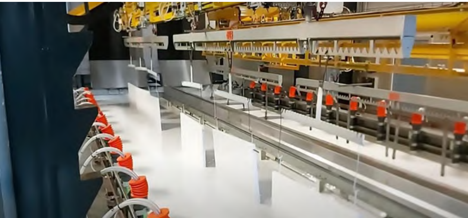
IN 2019, ZANARDO S.P.A, AN ITALIAN MANUFACTURER OF ELECTRICAL CONTROL CABINETS, INSTALLED A FULLY AUTOMATED COATING FACILITY WHICH COMBINES E-COAT AND POWDER COATING. UTILIZING OUR INNOVATIVE ELECTRON LB280 COATING, THEY BECAME THE FIRST COMPANY IN EUROPE TO OPERATE AN E-COAT LINE WITHIN THIS SEGMENT.
