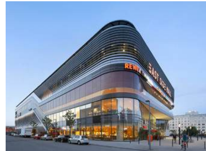
THE EXTERIOR OF EAST SIDE MALL BERLIN IS COMPLETELY COATED BY GRAVIHEL
